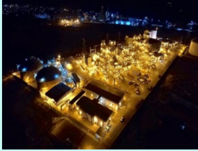
Kpone Power plant in Ghana (340MW)
