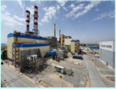
Rades-C Power plant in Tunisia (450MW)
