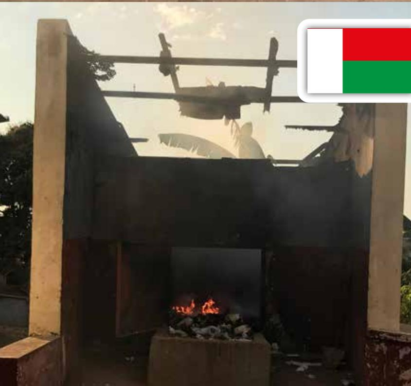
Current situation of the infectious waste incinerator at CHU Pzaga
