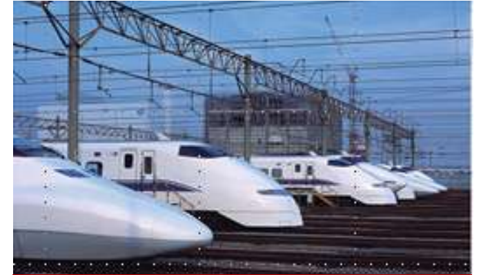
Railway Power Supply
