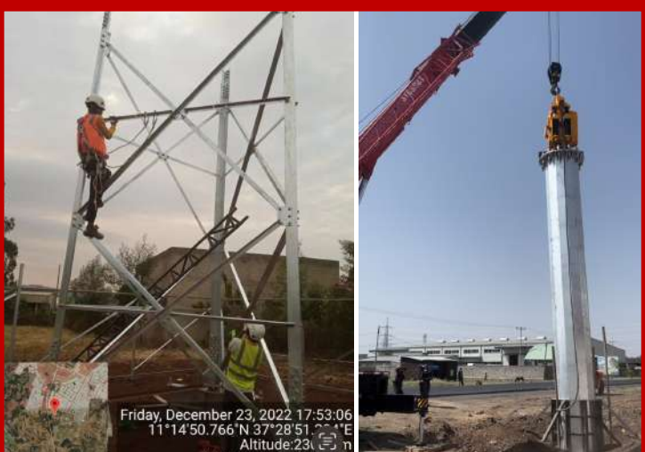
New Foundation Method Telecom Tower(with HUAWEI)
