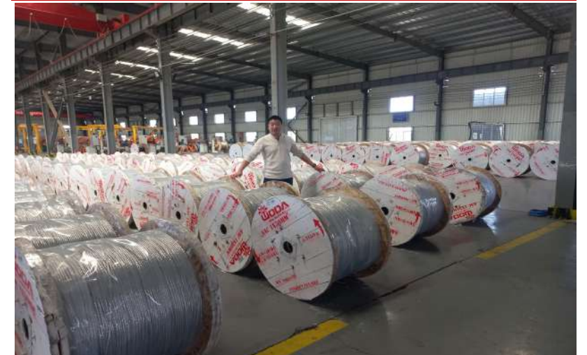
EEU 33/15KV Transmission Line 10KM
