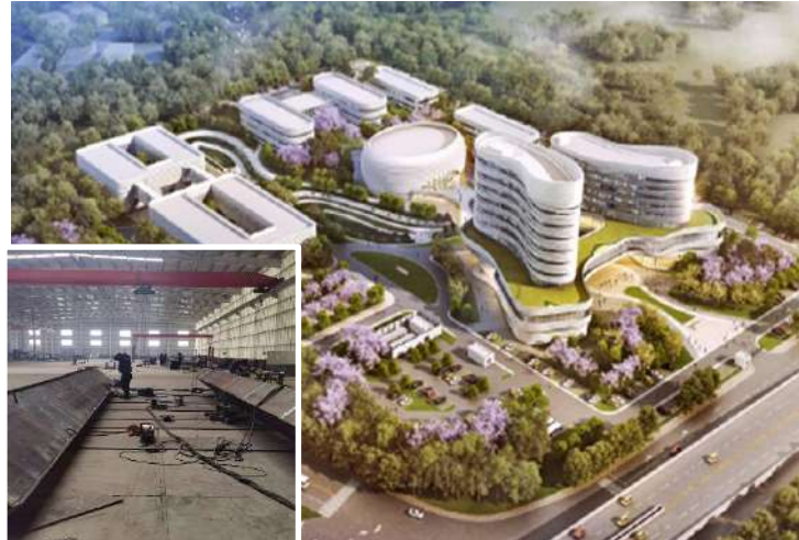
Embedment (African CDC project CCECC)
