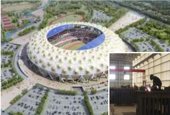
Embedment(ET National Stadium project CSCEC)
