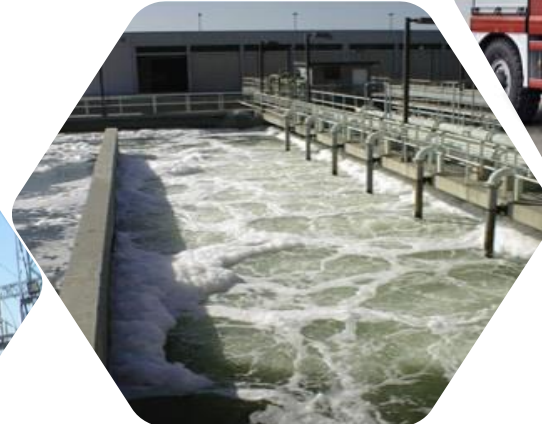
Water Treatment Facility (ZLD)
