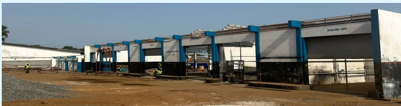
Ongoing Construction Work at GTI Kissy
