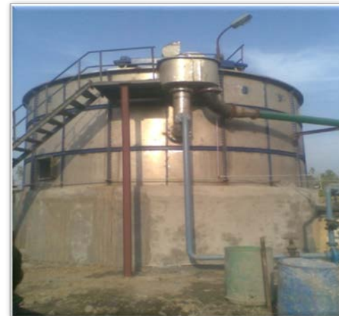
Installation of Fiber Recovery System
