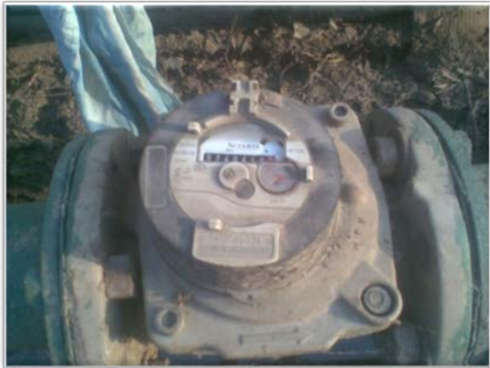
Installation of Borewell Flow meter/ Electronic Flow meter
