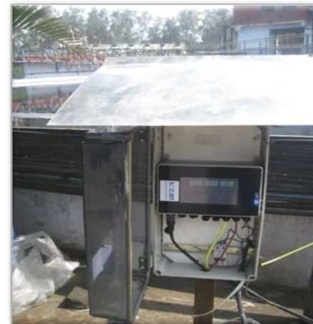
Installation of On line Monitoring system
