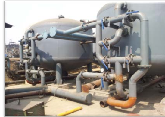
Installation of Tertiary Treatment System
