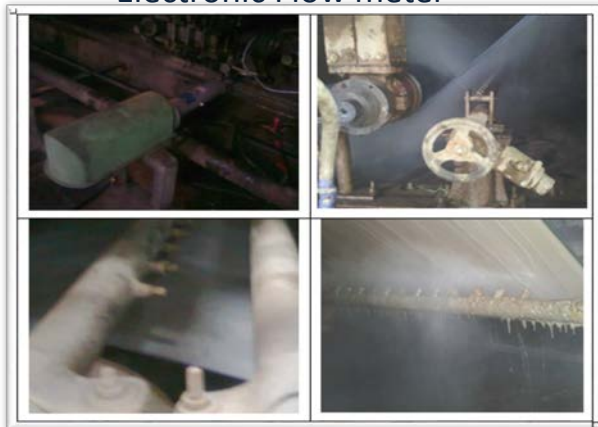
Installation of Paper Machine Showers of Specified Diameter
