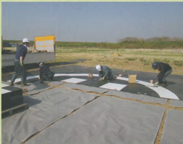
REPY BOARDs placed on the plastic sheets.
