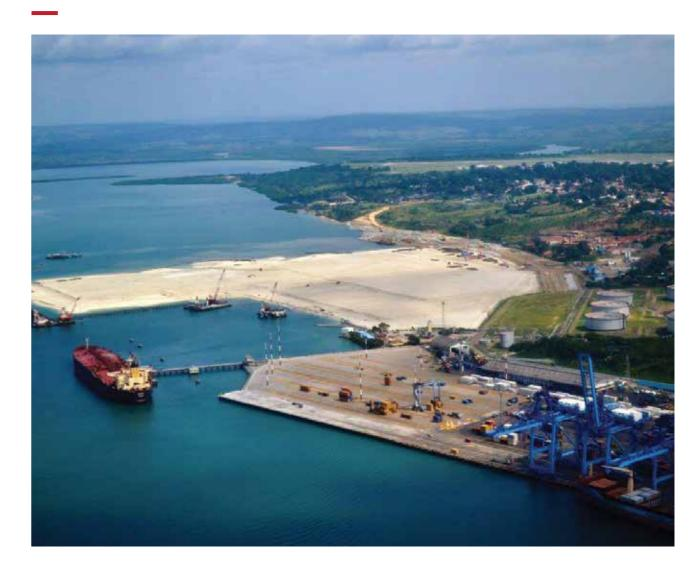
The Port of Mombasa is Kenya's principal seaport, comprising Kilindini Harbour and Port Reitz on the eastern side of Mombasa Island, and the Old Port and Port Tudor on the northern side. The main harbour is Kilindini, which is naturally deep and well sheltered. It has 16 deepwater berths, two oil terminals and safe anchorages, and mooring buoys for ships anchoring at sea.
