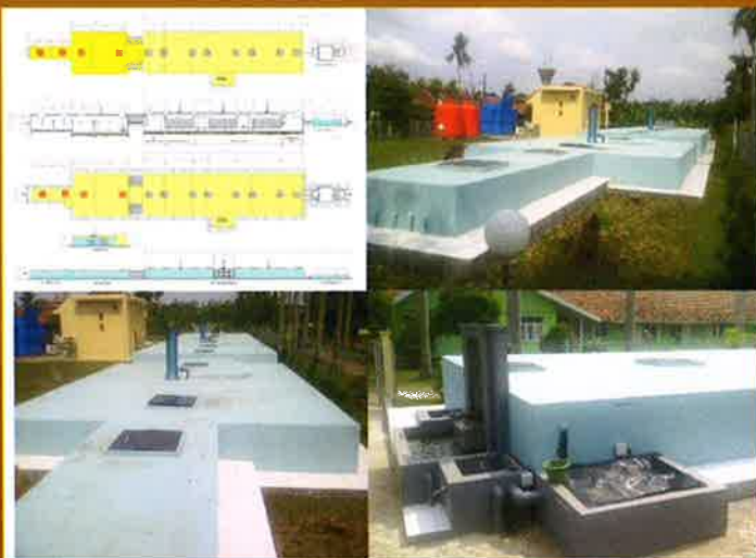
DOMESTIC WASTEWATER TREATMENT USING ANAEROBIC-AEROBIC BIOFILTER CAPACITY 200 M 3 PER DAY
