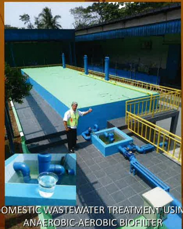
THE DIAGRAM OF DOMESTIC WASTE WATER TREATMENT USING ANAEROBIC-AEROBIC BIOFILTER PROCESS
